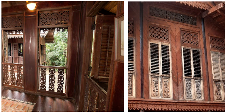
Figure 2. Openings aided by ornamentation at the serambi walls in Malaysia vernacular design buildings.
