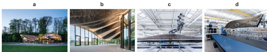
Figure 3. Hybrid Fiber Pavilion (a) Exterior view showing the undulating roof; (b) Interior view showing fibre bodies of the hybrid roof elements; (c) Robotic prototyping of component in research context; (d) Production winding of component in industrial context using conventional filament winding machine © IntCDC University of Stuttgart
