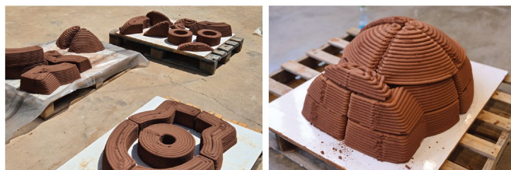
Figure 4. Assembly of the soil dome from the separately printed segments
